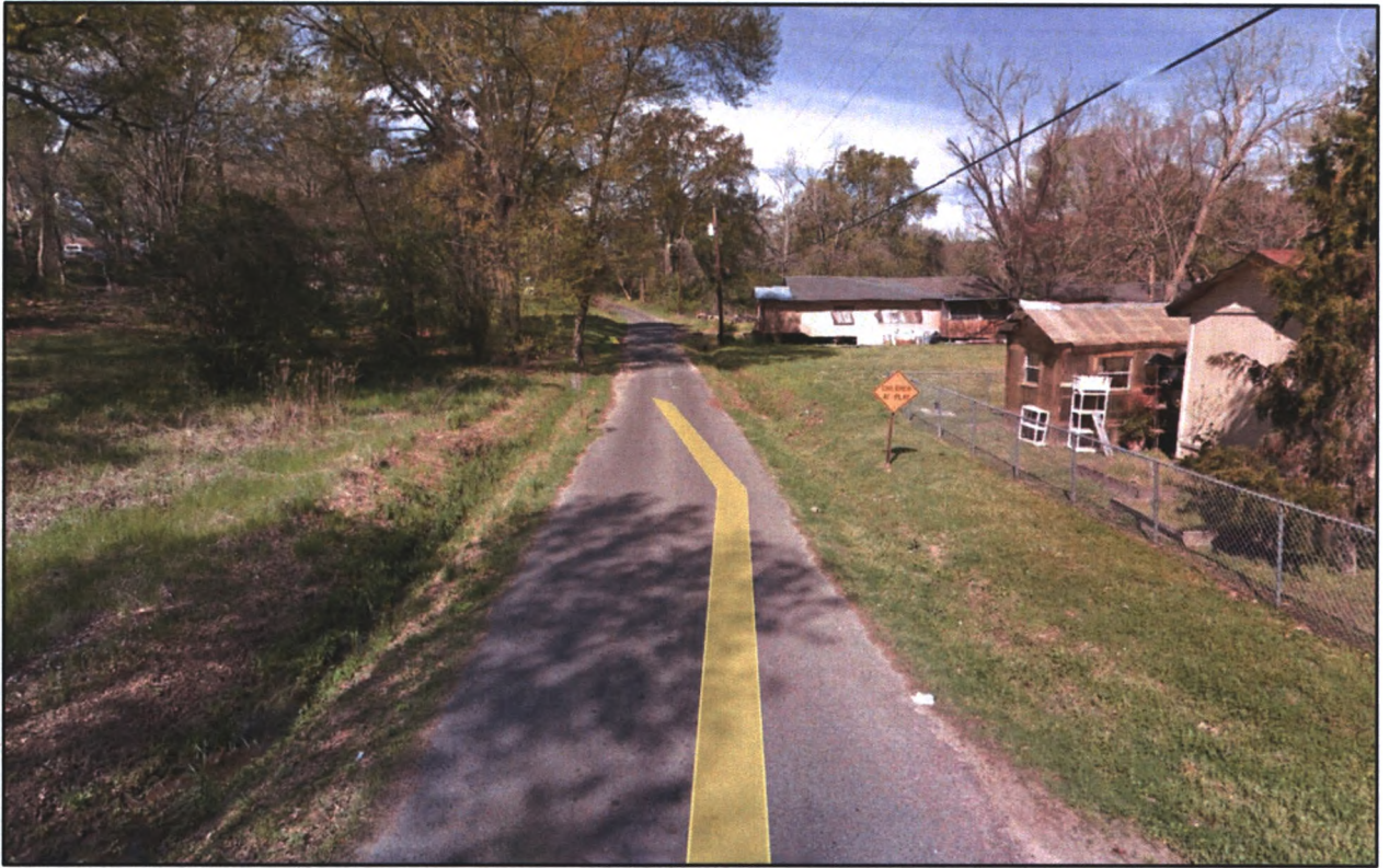
Figure 1.5 – Narrow Street & Shallow Ditches
