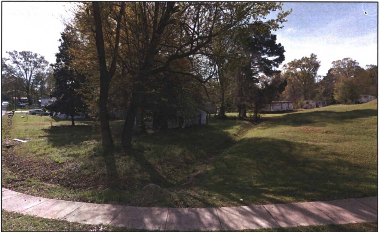
Figure 1.3 – Shallow Ditch Near Welch Street
