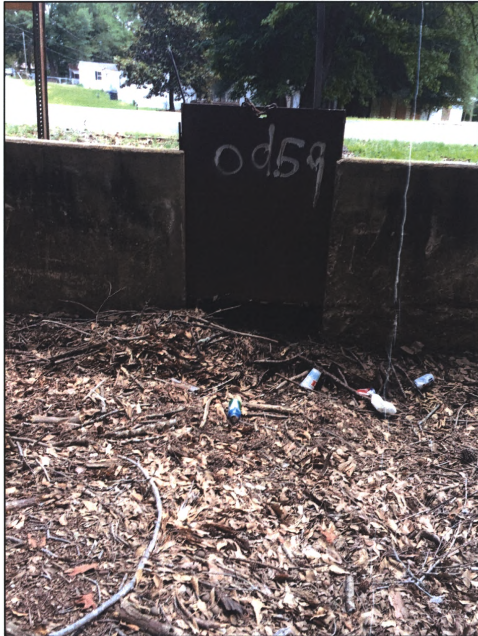
Figure 2.4 – Metal Sluice Gate Restriction
