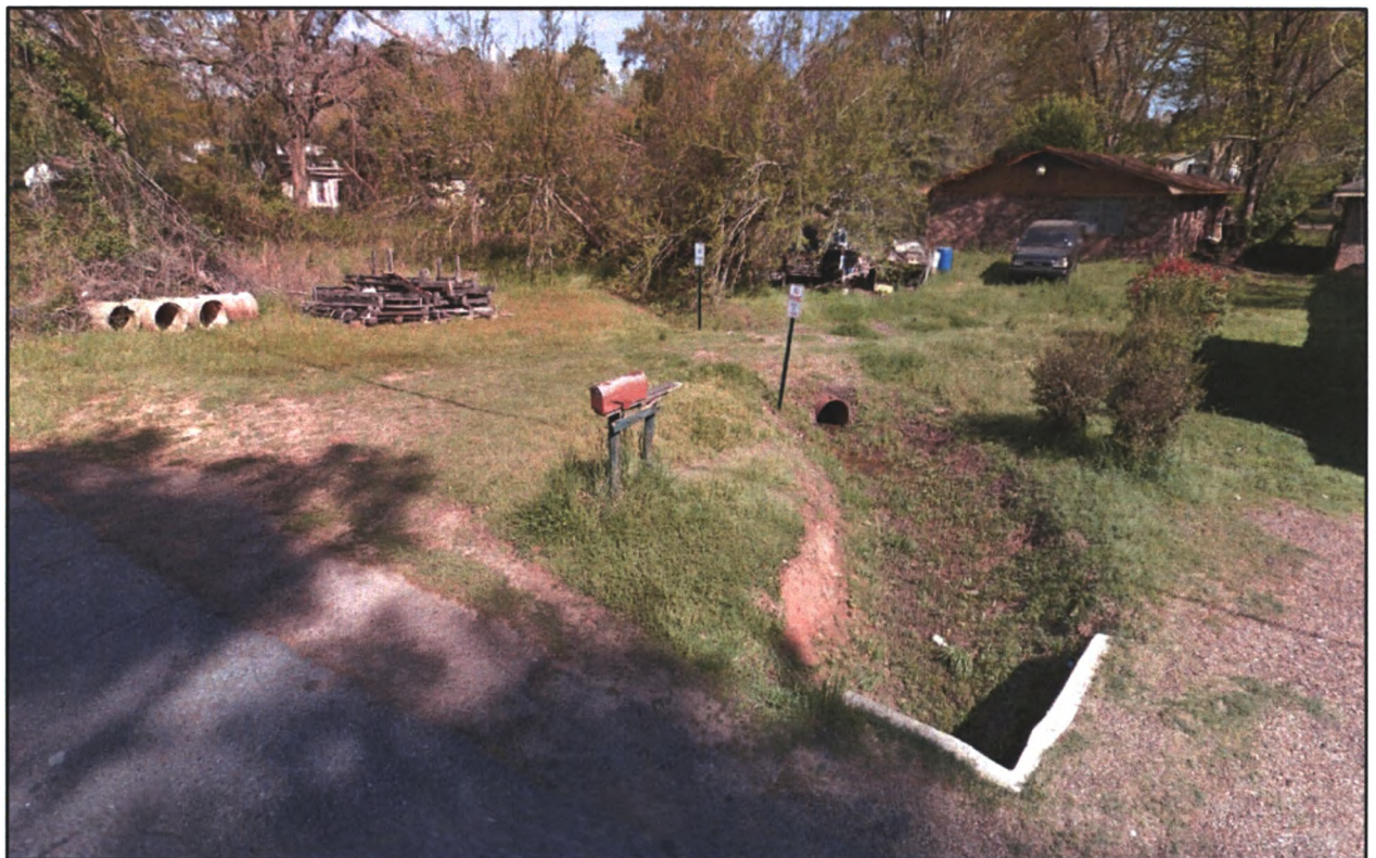
Figure 1.4 – Meandering Grownup Ditch
