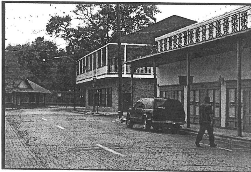
The building in the middle of this picture has good intentions, but the balcony should be supported by columns rather than being cantilevered.
