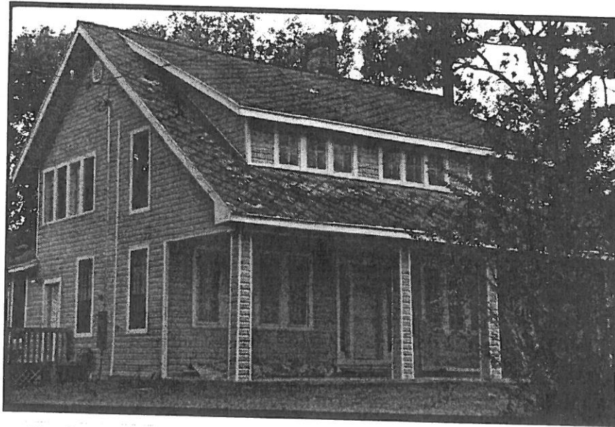
Vinyl siding alters the character of an historic structure. Note the inappropriate use of horizontal siding on the columns.
